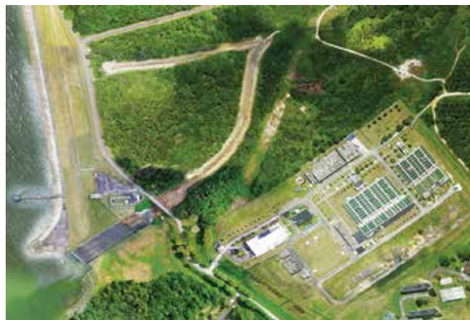
► Sungai Layang Dam is the catchment area for Sultan Iskandar WTP.
