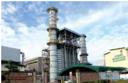
▶ Rugading Power Station, Sabah
